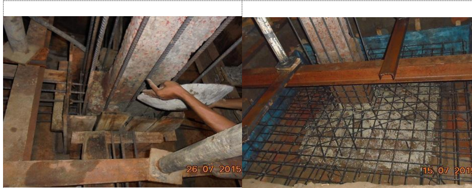
FIGURE: - RETROFITTING OF COLUMN DEA, (FAKIR TEXTILE MILLS, NORSHINDI)
