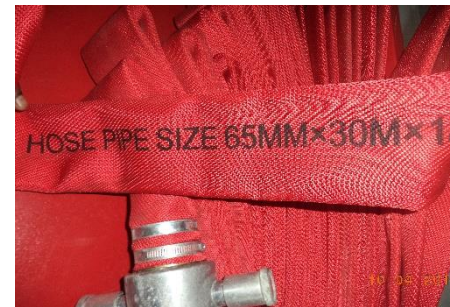
FIGURE: - HYDRANT SYSTEM TEST
